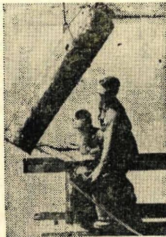
**TOPPING OFF . . .** Using precision of a ballet team, two Navy Seabees saw the excess off lengthy piles in process of bridging a Vietnamese River.
