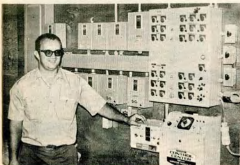
FANCY WIRING —Bob Neldinger, of Sam's Electric in Culver, designed this special wiring, which automates the dairy feeding operation. Through special stepped controls all feed storage bins, all Harvestores, augers, and additive mixers can be controlled from one location, without danger of system clogging.
