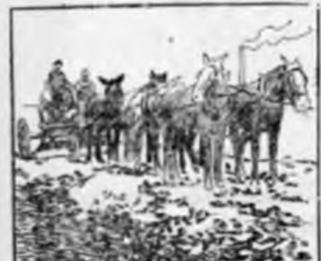
Slag Foundation and Broken stone Surface.
