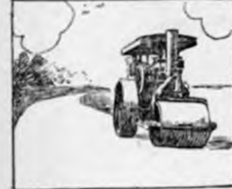
Steam Roller Finishing the Surface.
