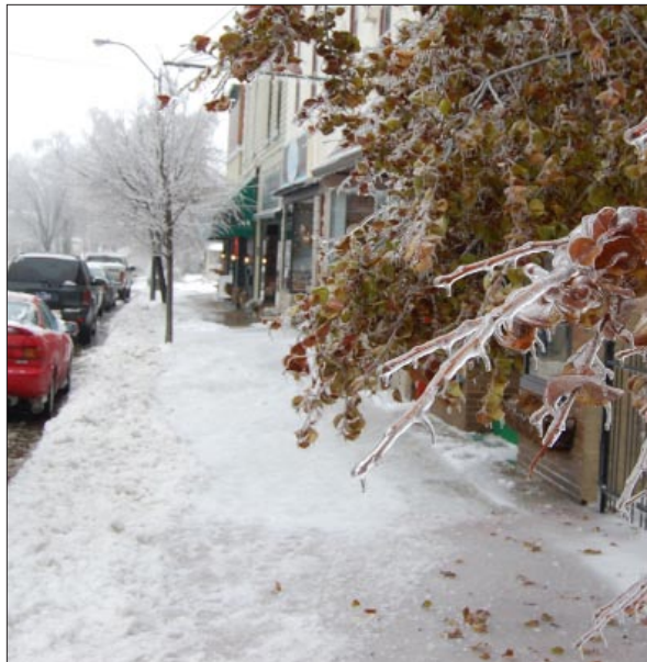
Downtown sidewalks are generally some of the clearest in town, in spite of the thin coat of ice in this December, 2008 photo. Some Culver residents are concerned about the safety of many of the town's sidewalks during the fall and winter.
