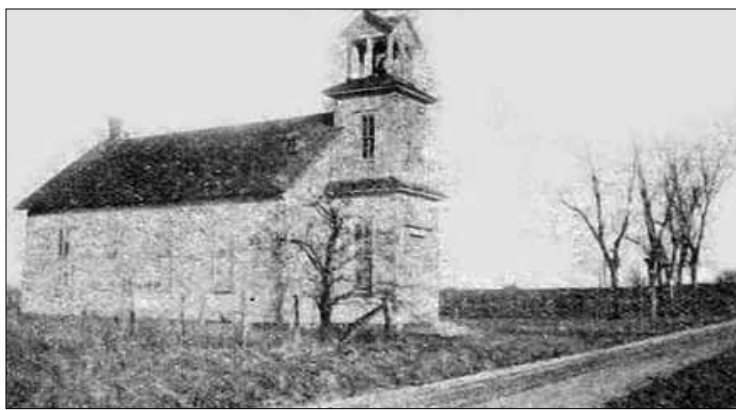
The Washington Evangelical Church in days gone by, prior to its 1939 demolition.
