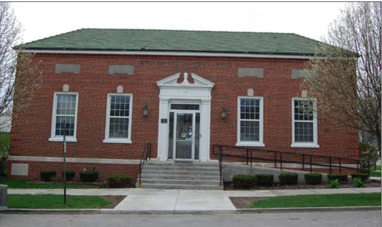
ABOVE: Culver's 1935-built post office, at 115 W. Jefferson Street near downtown.
